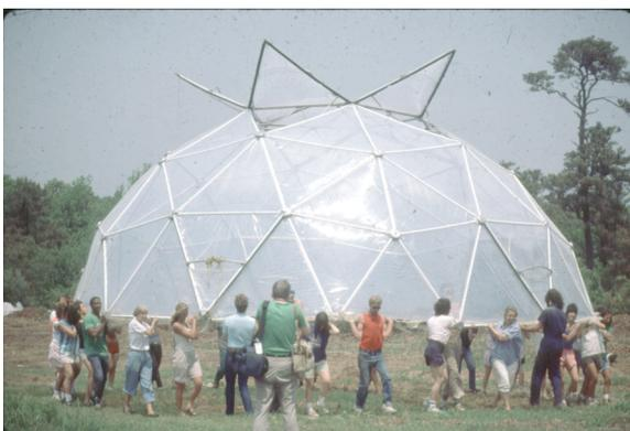
When the 1 pillows are inflated, the entire dome is put under compressive load that tends to oppose the considerable wind lift. This preloading, together with the anchoring provided by buried concrete blocks tied to the lowest hubs, has withstood 30 inches of snow load and winds well above 100 mph. This may be considered good performance from a structure that weighs but 1/2 lb/ft<sup>2</sup> of floorspace (less than 500 lbs total). The light weight not only results in low shipping
