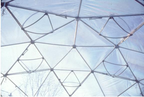
The physical performance has been good. The biological performance has equaled the original New Alchemy Ark in output per square foot, that is, commercial production quantities. Moreover, the pillow dome's natural air circulation patterns have eliminated the need for that nuclear fan. The dome also casts but 1/5th the shadow of a more conventional greenhouse, important for winter growing.
